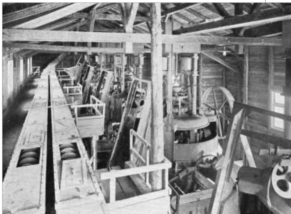
Figure 9: Mixing station in the construction of the Kiel Canal (1907 to 1914)
