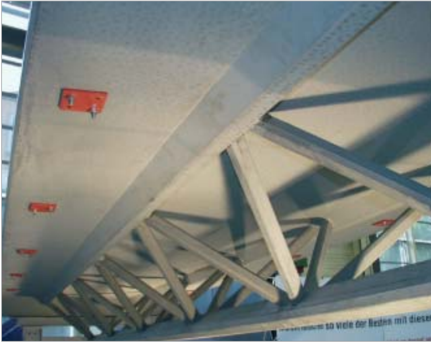
Figure 23: Bridge section made of Ultra High Performance Concrete, produced by Max Bögl, Neumarkt, Germany
