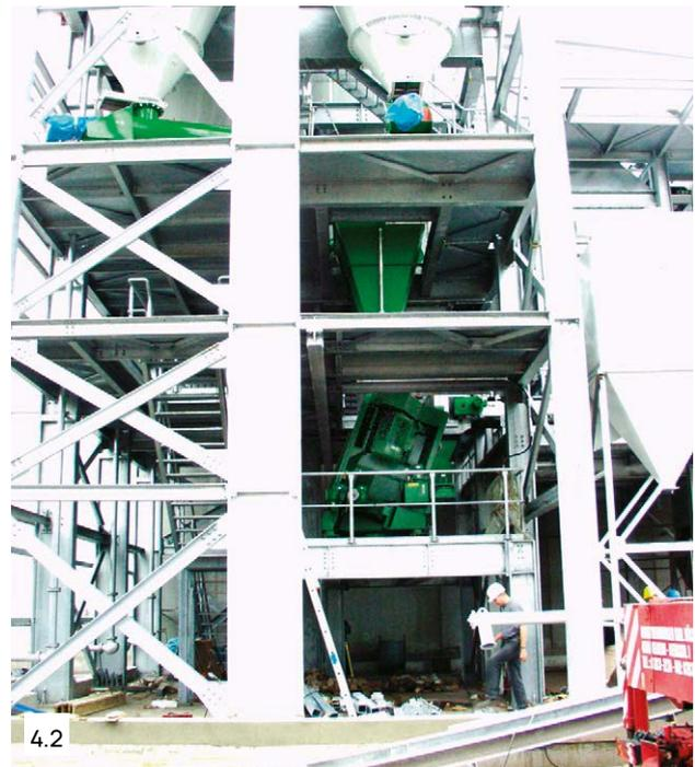
Fig. 4.2: Assembly of the continuously operating agglomeration system
