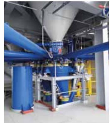
R12W intensive mixer, lift and swivel hoist      Silos and scale
